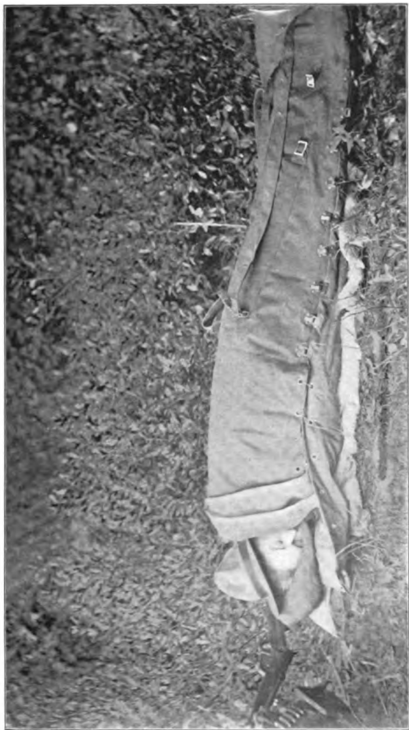
PACK SACK SLEEPING-BAG DESIGNED BY THE AUTHOR. The picture illustrates how the bag is fastened in use by bronze army snap-hooks
