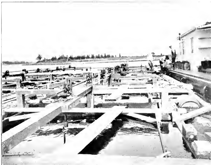
FIG. 7.—Starboard side, looking aft, inside float. Shafting system and general arrangement of cars.
