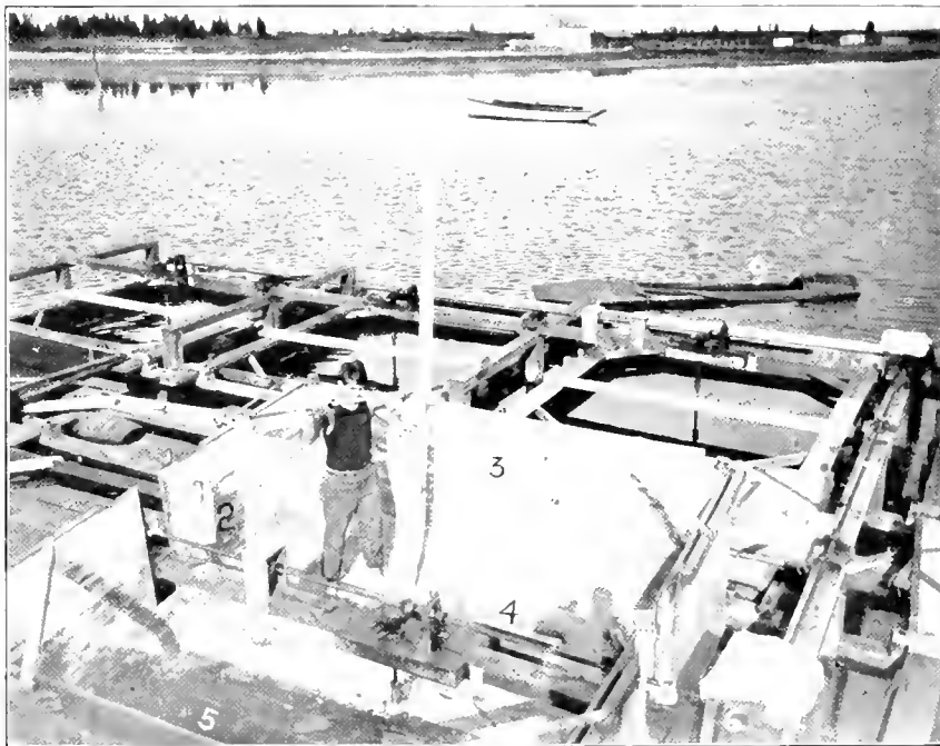
FIG. 6.—Interior of rearing car, and propeller. 1, slot in end of car, 2, doors for closing the slot; 3, side screen windows; 4 and 5, bottom windows; 6, box covering gear trains, 7, transverse shaft, 8, longitudinal shaft, 9, towing car. The arrangement of shafting on latter float can be seen.
