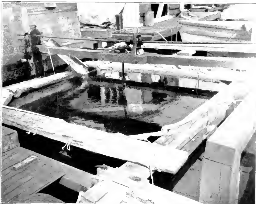
FIG. 16.—Filter car with canvas lining. Chain buckets on left. The propeller blades may be seen in the water.
