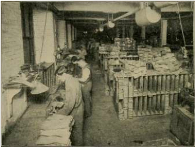
The Cut-Sole Room in the Shoe Factory
