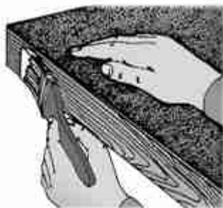
FIG. 13 - After applying two coats of cement to edges, apply one coat to back of laminate.
