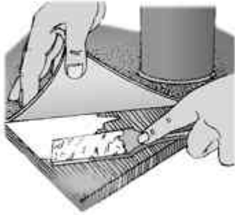
FIG. 7 - You can use a handmade wood paddle for spreading the contact cement
