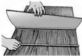
FIG. 9 - On large areas, longer dowel rods are needed to hold the laminate away from the cemented surface.
