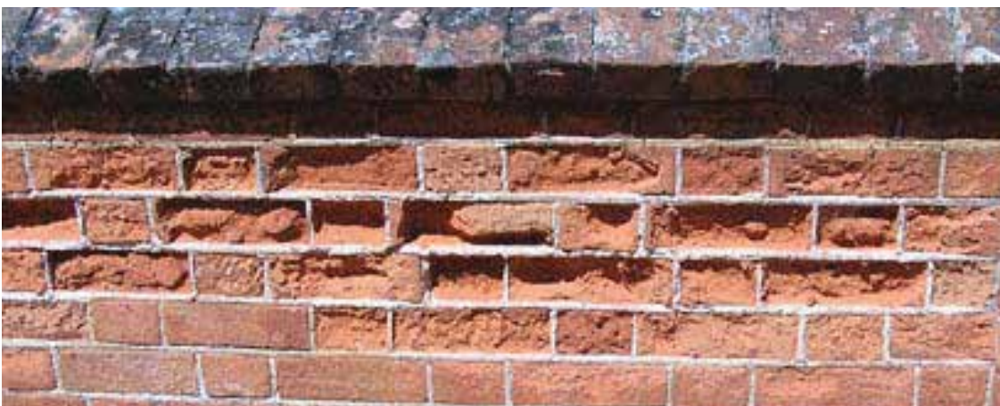
Figure 3 – Effect of salt attack on brickwork
