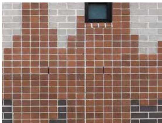
Figure 5 – Control Joint
