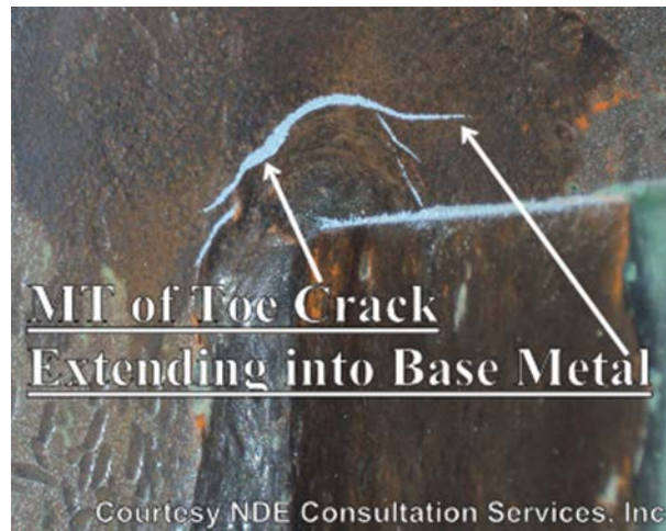
Figure 21: MT of toe crack
