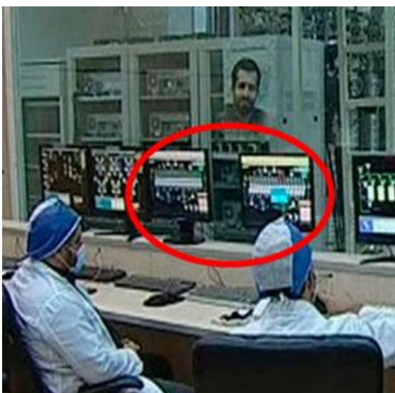
Figure 5: Operators in front of the SCADA displays of the Cascade Protection System, placed right below a picture of former president Ahmadinejad
