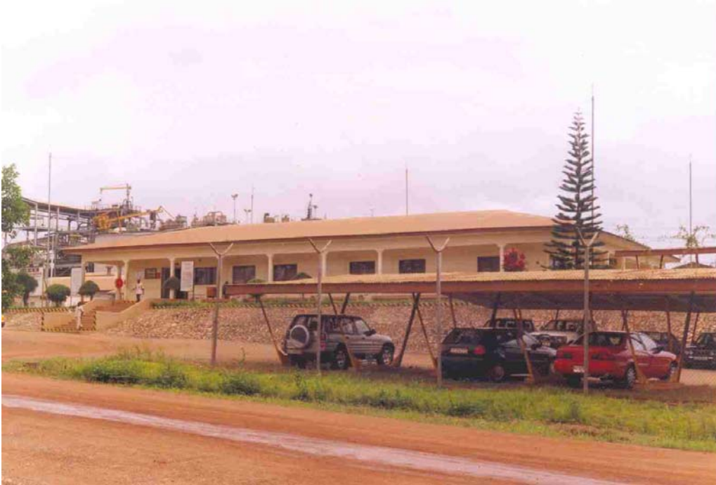
Figure 6: Front View of Administration Building
