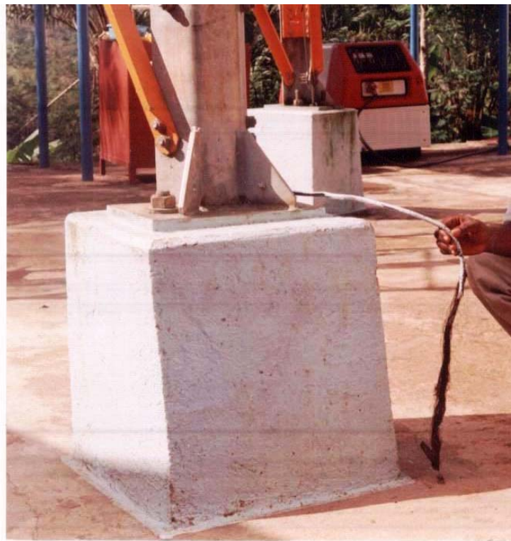
Figure 10: Bunt insulation of the tower down conductor
