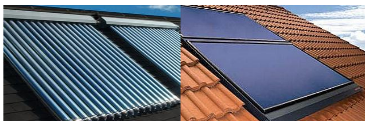
Figure 7-1 Solar Thermal Panels: Evacuated Tube & Flats Plate Panels
