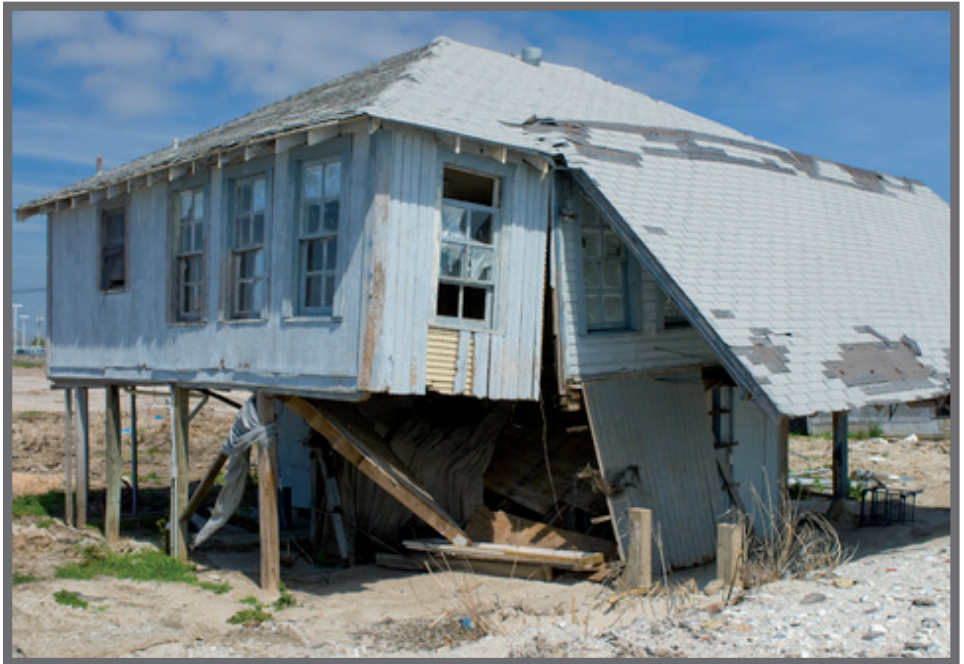
Aftermath of Hurricane Katrina
