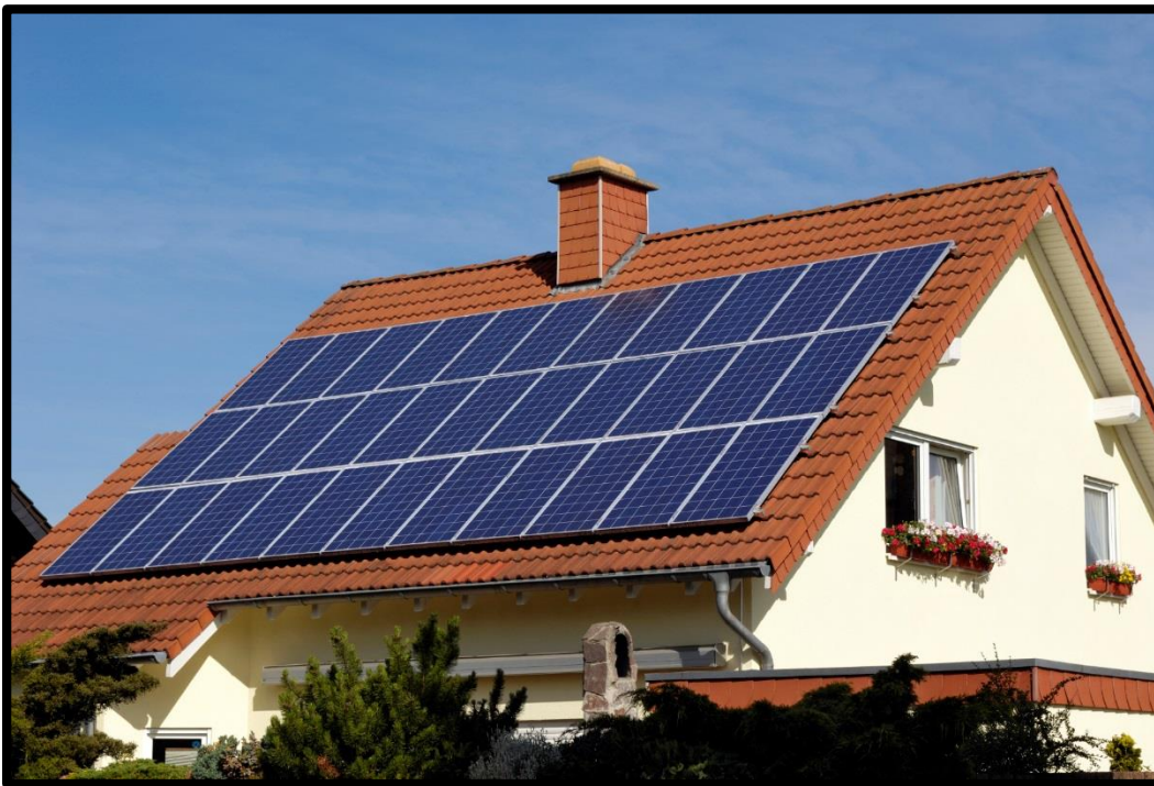
SOLAR SYSTEMS ARE GETTING LESS EXPENSIVE AND MORE EFFICIENT ALL THE TIME.
