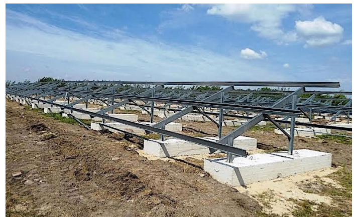
PV support structure and concrete foundation ( Hill & Smith )
